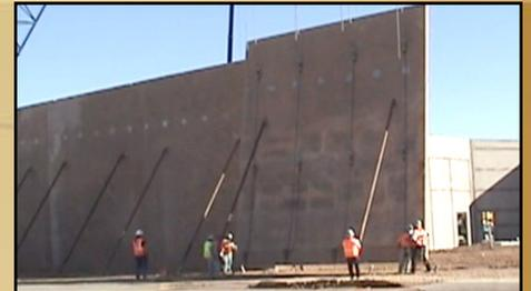
The newly developed Insta-Brace Anchor by PierTech Systems provides tilt-up contractors with an economical and efficient alternative to cast-in place, concrete dead-man.
