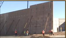
The newly developed Insta-Brace Anchor by PierTech Systems provides tilt-up contractors with an economical and efficient alternative to cast-in place, concrete dead-man.
